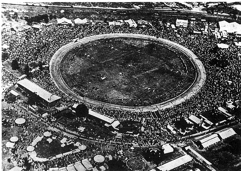
Aerial view of the Claremont showgrounds 1934
